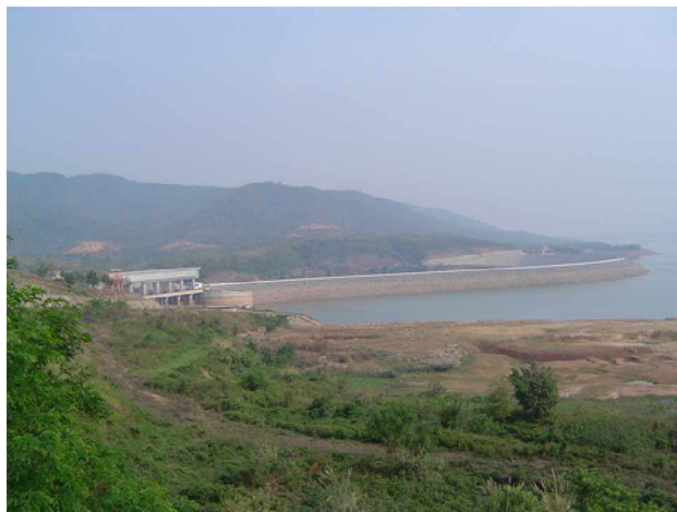
Yaly Hydro Power in Gia Lai province
