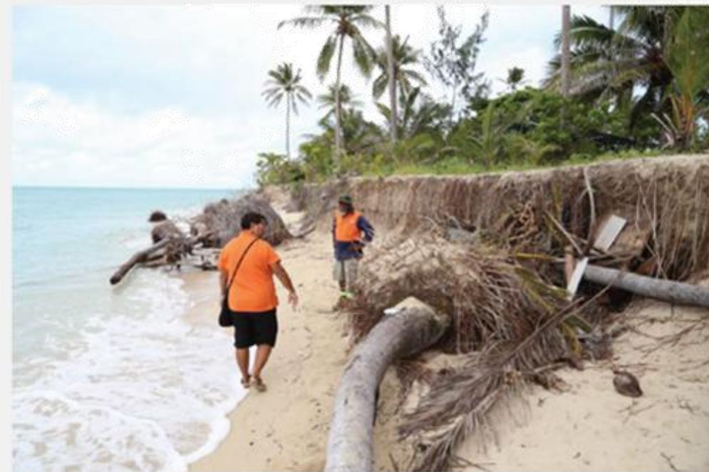
Poruma Island local, Olandi Pearson, shows Mary Bani (TSRA) severe coastal erosion, a source of great concern to the inhabitants of this remote coral cay. Photo: John Rainbird
