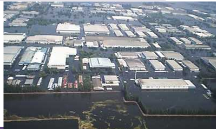
Flood in Rojana Industrial Park (Thailand, October–November 2011) Source: Basic knowledge on flood control, the Ministry of Land, Infrastructure, Transport and Tourism
