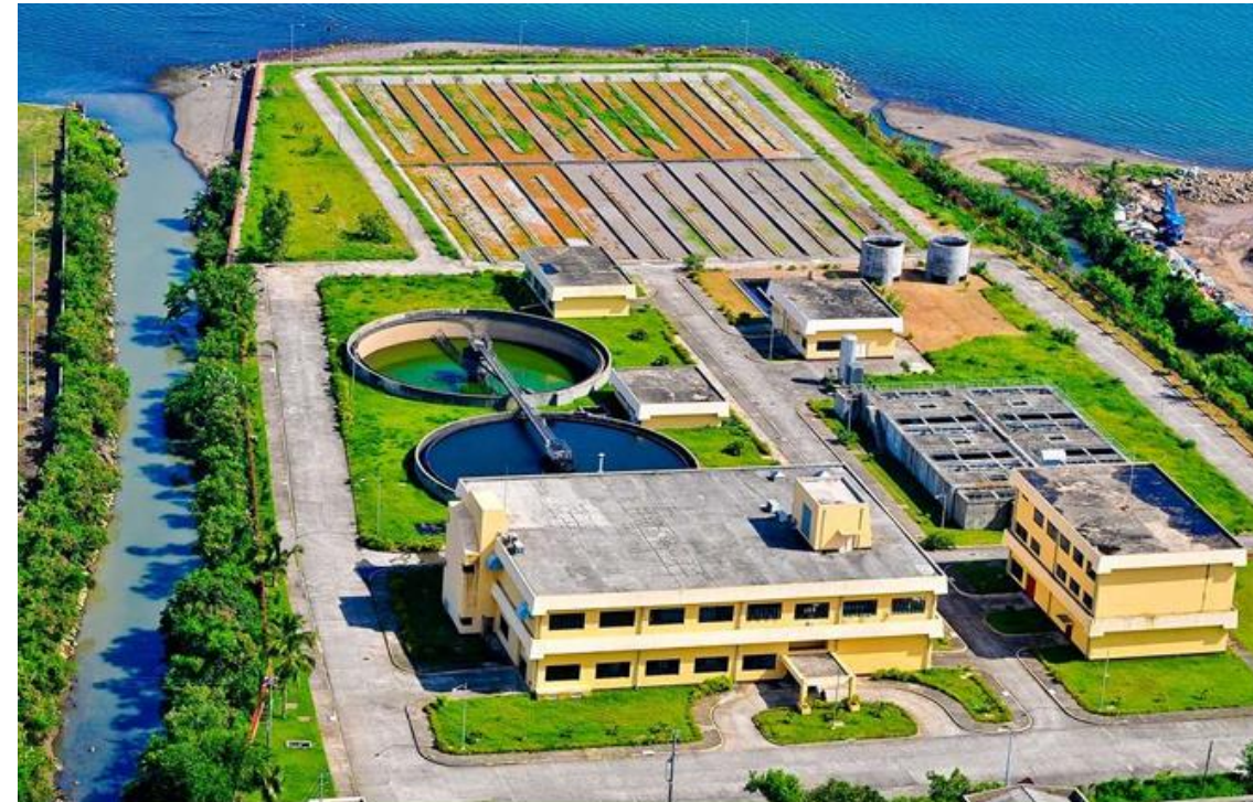
Wastewater Treatment Facility of the Authority of the Freeport Area of Bataan (AFAB) located in Mariveles, Bataan
