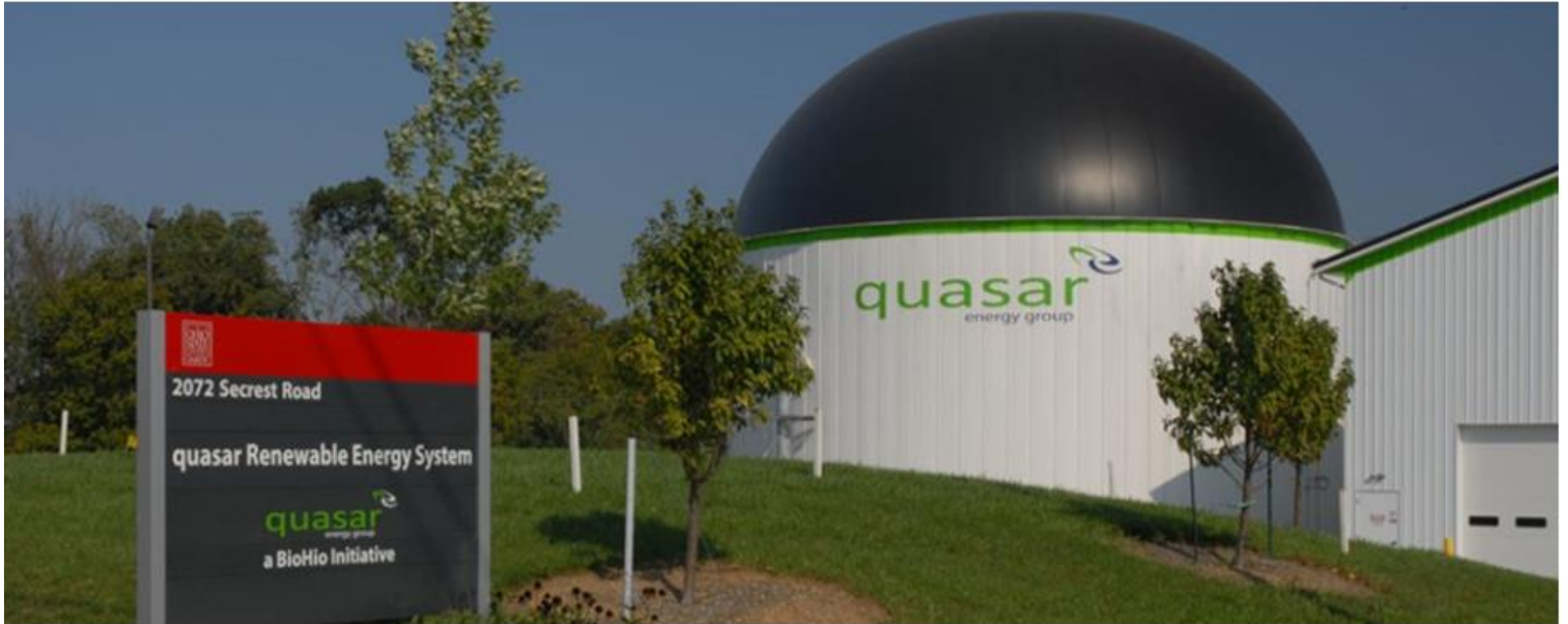
Anaerobic Digester in Wooster, Ohio
